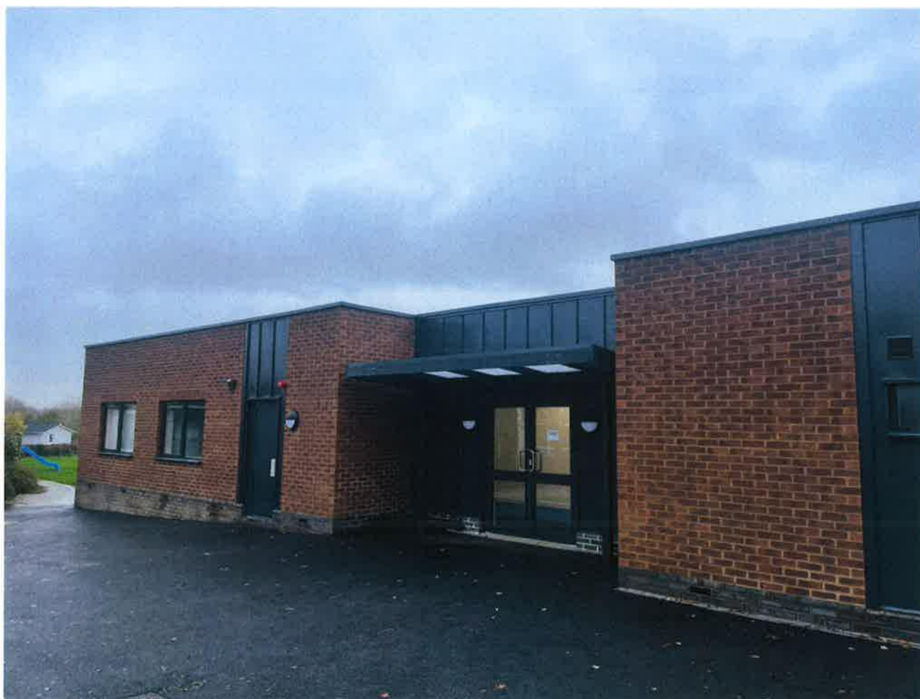
John Wycliffe Primary School modular build
