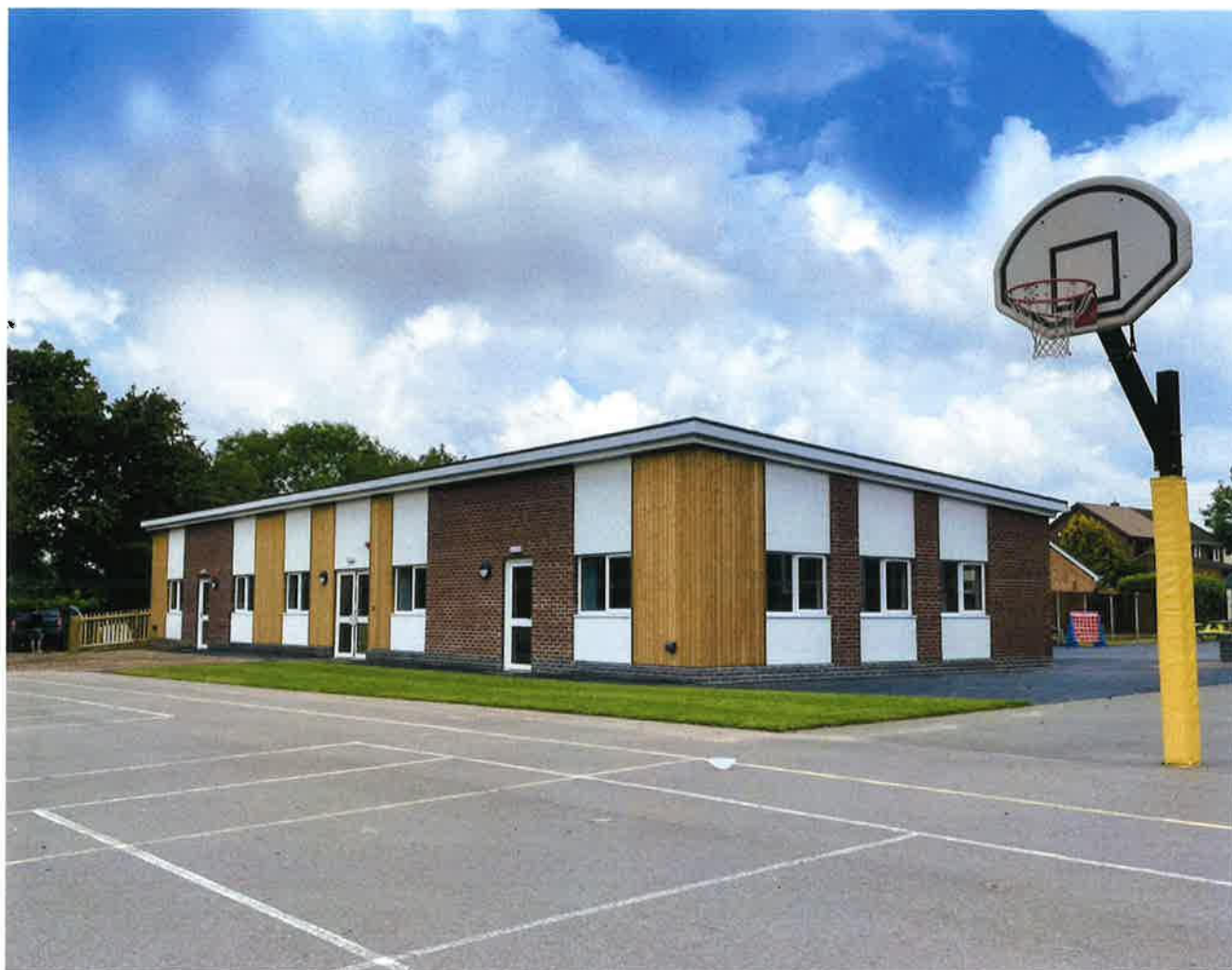
All Saints CE Primary School Sapcote phase 5 modular build (picture courtesy of YMD Boon)
